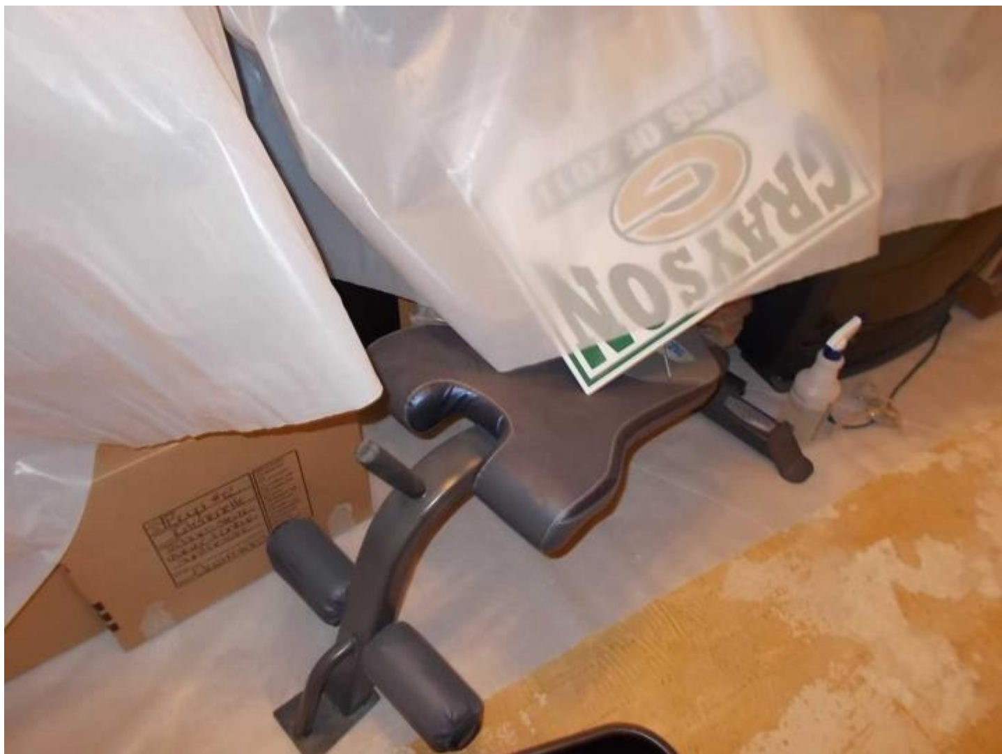
14 DSCN0014 Date Taken: 3/12/2015 Taken By: George Niezgoda GLue on floor in main area giving off VOC's and causing discomfort to home occupants.
