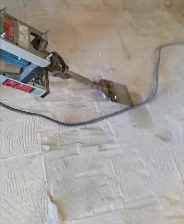
On or about 4/28/2015; Instrument used by Servpro to remove tile floor
